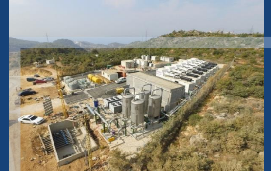
HANDLED SCOPE: EPC AND O&M OF THE LANDFILL POWER PLANT
