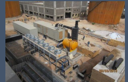
CONTAINERIZED GENSET CONFIGURATION
