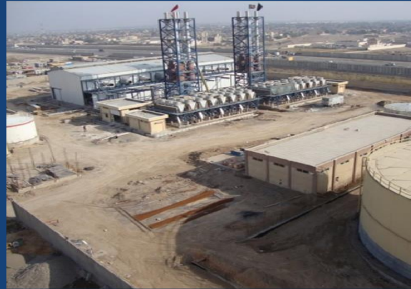
ELECTRICAL OUTPUT: 62MW
